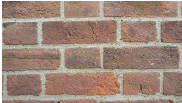
FIGURE 25: EXAMPLE OF NEAT MODERN POINTING, REGULAR JOINTS WITH THE EDGES OF THE BRICKS CLEARLY DEFINED
