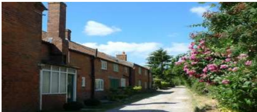
FIGURE 11: ROWS OF FORMER AGRICULTURAL WORKERS COTTAGES INTEGRATED WITH LARGER PROPERTIES ON LONG LANE
