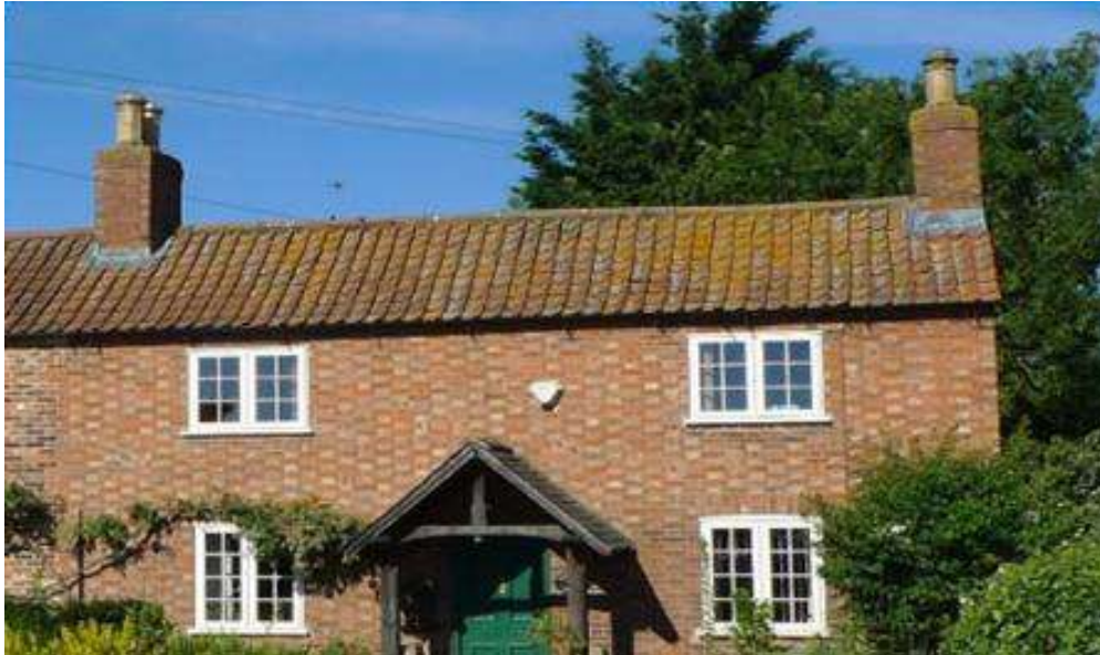
FIGURE 16: EXAMPLE OF A PANTILE ROOF
